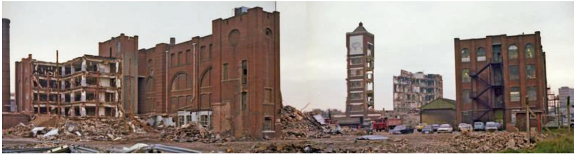
Fig 8 Demolition of the Orchestrelle works in 1976
