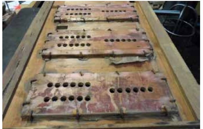
Fig. 9 Rusted screw holes, split valve boards, and open glue joints
