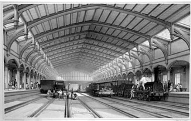
Fig. 11A. The engine shed of Brunel's Temple Meads station, 1843, showing the 7 foot broad gauge tracks and engines.
