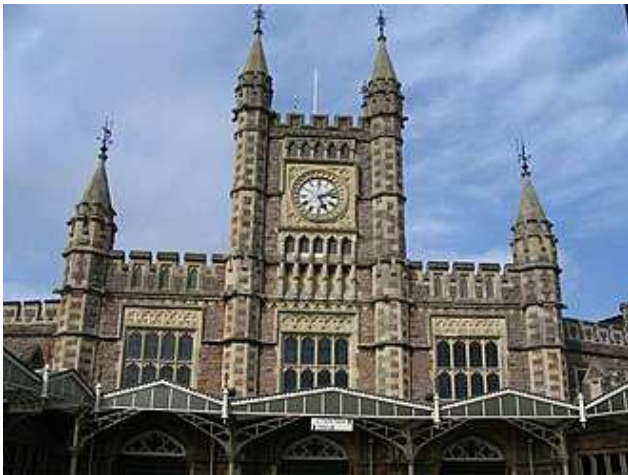
Fig. 11B. The station façade (Fig. 11A) remains much the same as Brunel's day but it had a spire that was removed before WWII.
