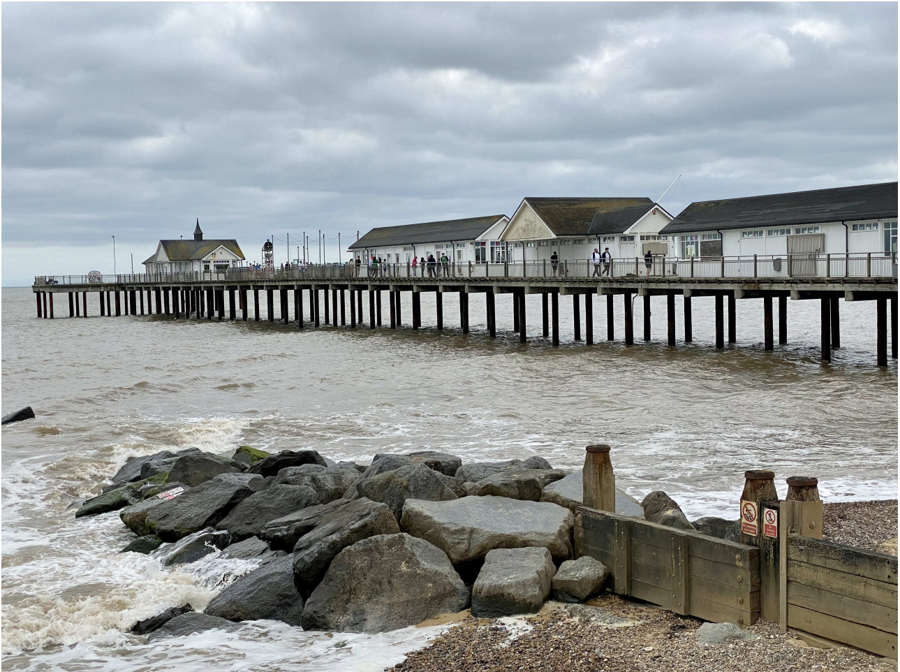
Photo 1: Southwold Pier, housing the 'Under the Pier' show
