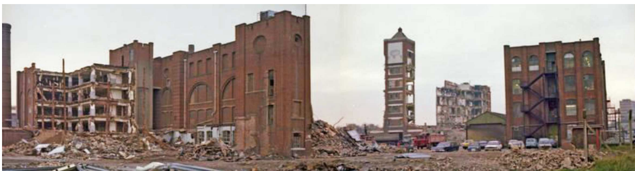
Fig 8 Demolition of the Orchestrelle works in 1976
