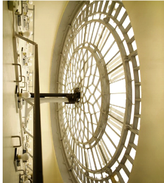
Fig 4. Electric lighting for the dial
